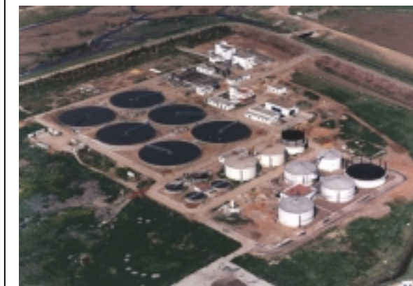
Water & waste treatment plant, Copero, Sevilla
