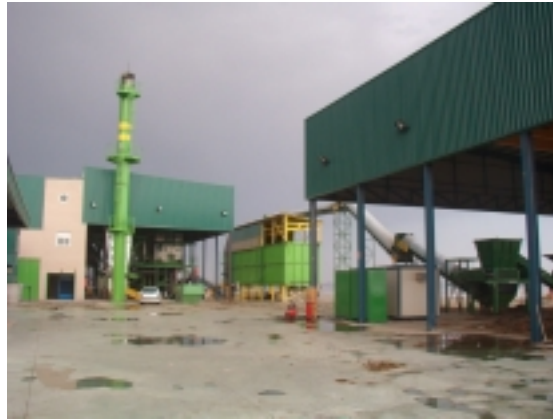
Gasification Plant at Níjar, Province of Almería
