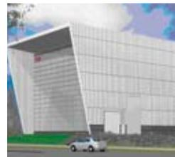
Lextorp CHP is a new biomass combined heat and power plant in the town of Trollhättan in Västra Götaland, Sweden. The design of the building is aesthetically pleasing and the plant well visible for all car passengers and drivers entering Trollhättan from the South. The plant has a total capacity of 21 MW, with 3.65 MW<sub>el</sub> and 17.4 MW<sub>th</sub>.
