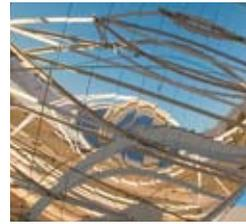
Andalusia is a pioneer in the research and development of high performance solar thermal power plants. Such a plant consisting of 624 heliostats with a surface of 121 m<sup>2</sup> each was installed in Sanlúcar La Mayor, Seville. It has a central receiving tower using saturated steam as working fluid. The nominal power is 11 MW<sub>el</sub> with an annual electricity production of 24.2 GWh.
