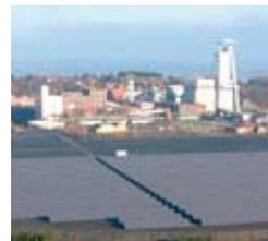
The world's largest solar PV-power station is located in Saarland. On a surface of 165.000 m<sup>2</sup>, 50,000 solar modules with a total capacity of 8.2 MW were installed on a former pond of an old colliery. The power plant was completed in 2005 and it produces electricity for about 3,400 households. The location in Saarland was chosen because of the relatively high solar radiation in the South-West of Germany.
